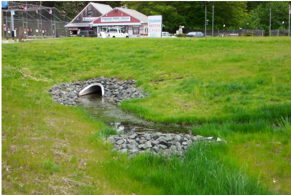
Example of grass lined channel stone dike/check dam
