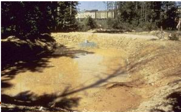
Example of Sedimentation Basin
