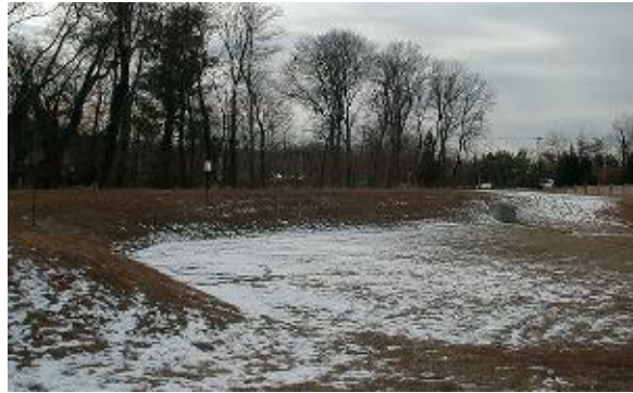
Example of Dry Extended Detention Pond
