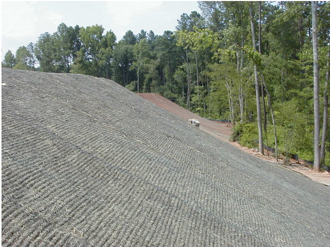
Example of Erosion Control Matting used for Slope Protection
