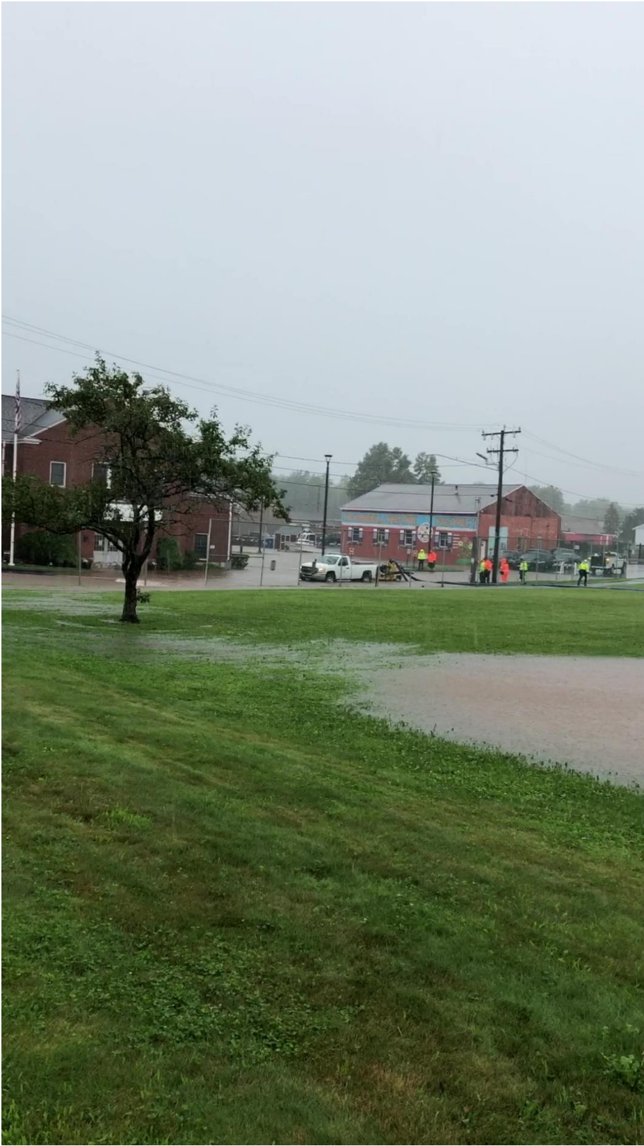
Culvert at Pierson Park Photo 2 of 4, photo taken 07/09/2021
