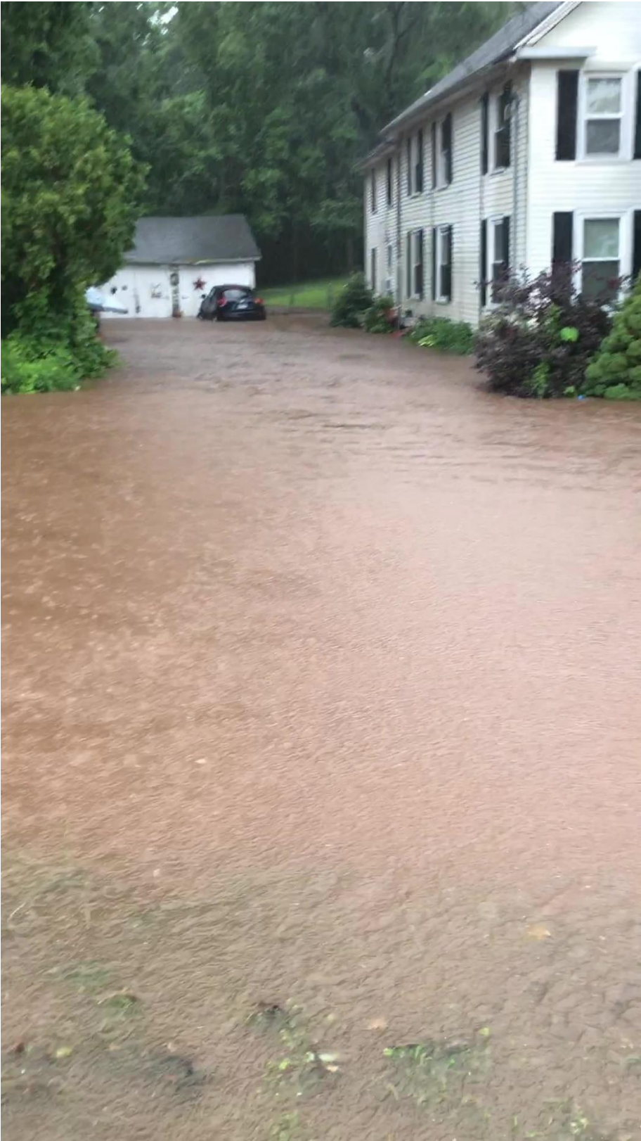
Culvert at Pierson Park Photo 4 of 4, photo taken 07/09/2021
