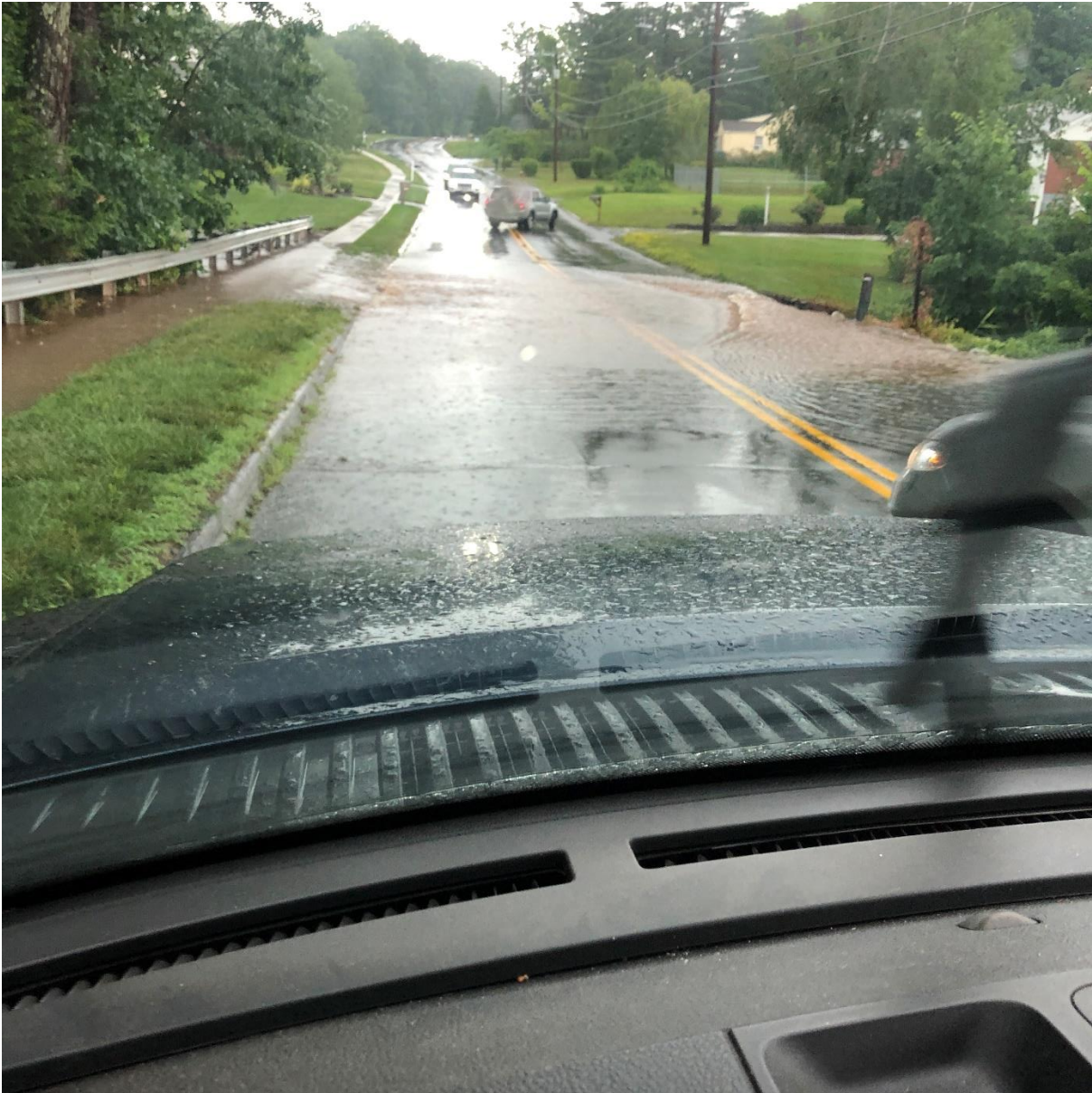
Willow Brook Cross Culvert- Evergreen Road, photo taken 07/09/2021
