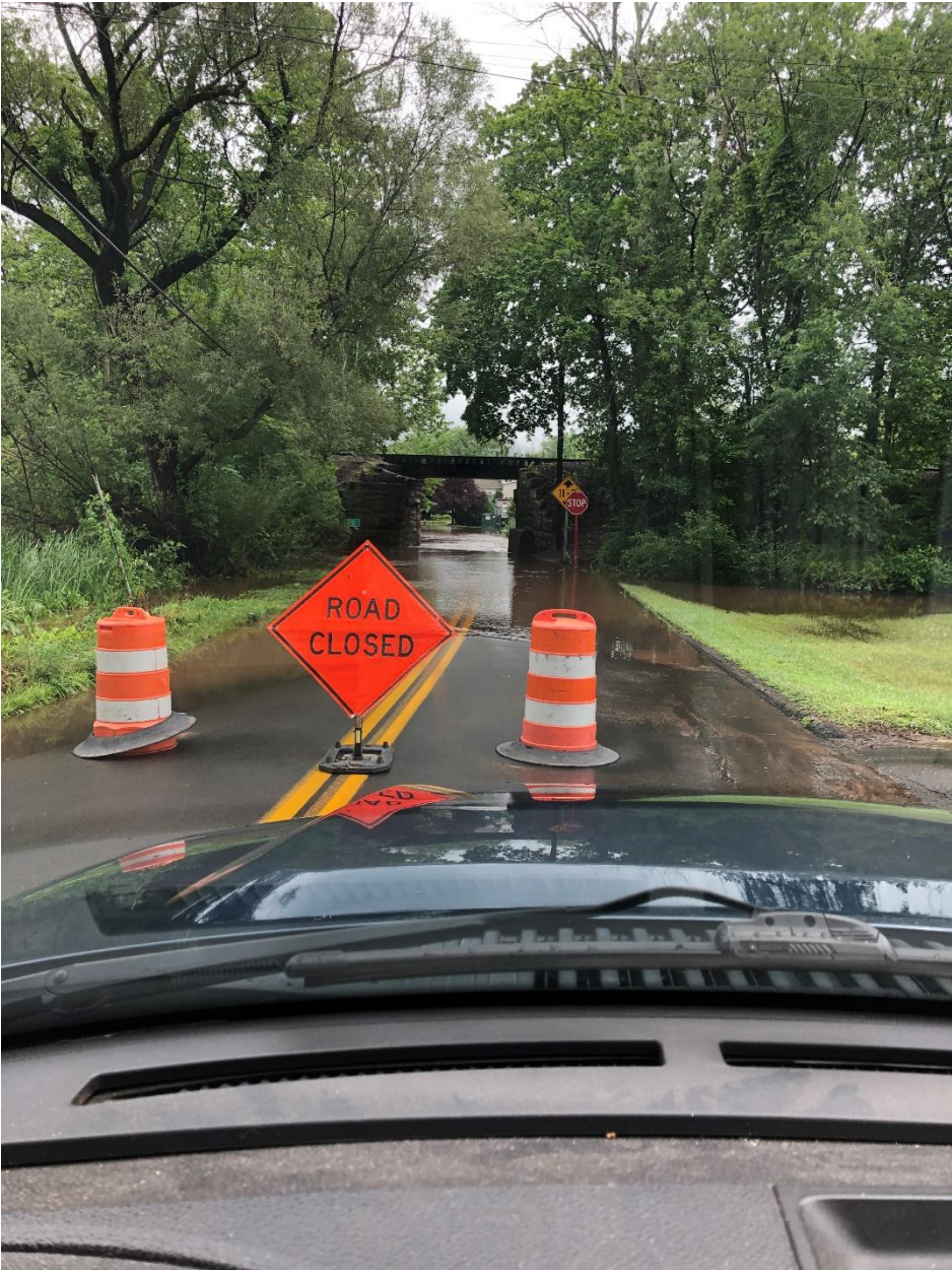
Culvert at South Street/ Railroad Trestle, photo taken 07/09/2021
