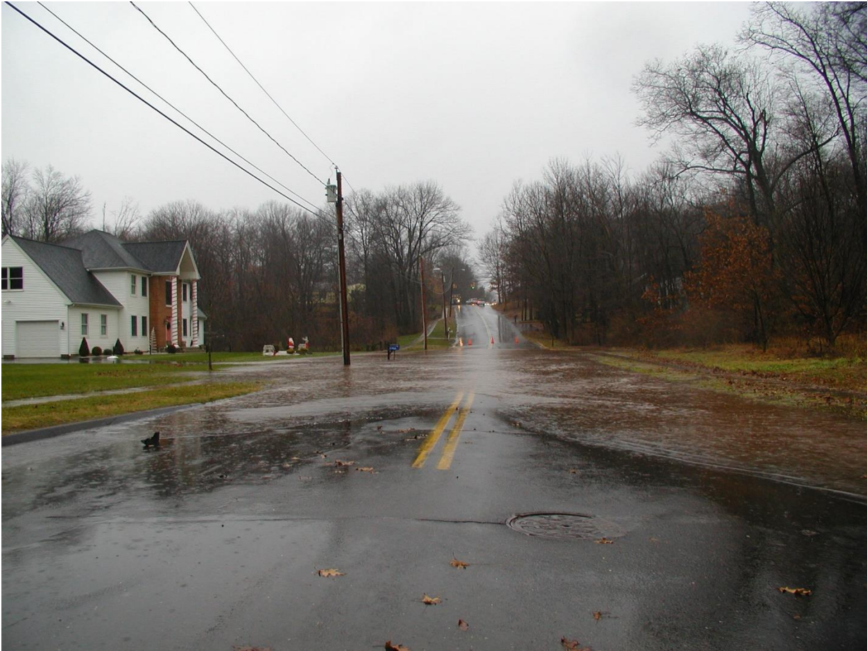
Culverts at Evergreen Road and Copper Knoll Drive, photo taken 12/20/2002
