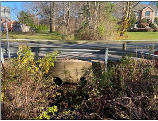
Downstream side of 18 & 24 inch RCP pipe culverts
