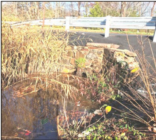
36 inch RCP outlet with brownstone endwall
