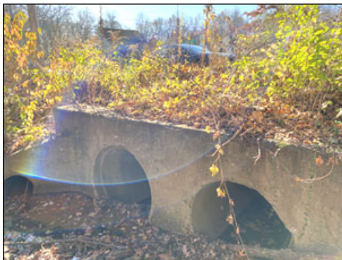
Copper Knoll-upstream side (twin 36-inch RCP)
